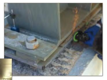
Anchor bolts were also isolated from any contact with the epoxy grout using PE foam and duct tape, to allow its stretching while tightening them.
