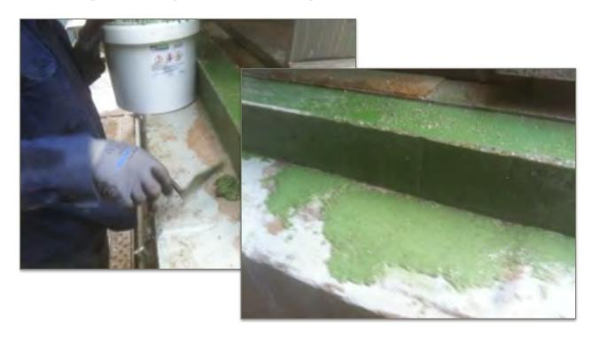
After taking off the pressure on the alphapads, the whole of the tank weight rested on the epoxy grout.
