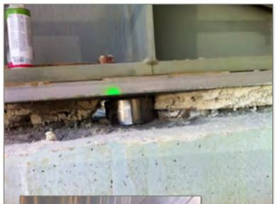
We centred our first efforts on the footings facing south. Using pneumatic chippers, we got rid of enough material form underneath the sliding plate to be able to place the first Alphapad sized D2. The quantity of material removed was sufficient to ensure a proper levelled surface with healthy concrete, and not enough to change in any way the position of the saddle.
