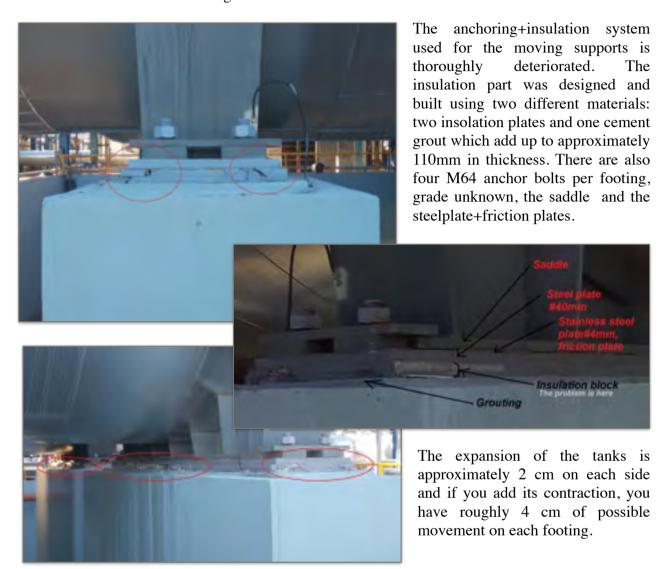
Assuming a friction coefficient for a steel-steel interface  $\mu$ =0,7 (usual values in between 0,5 y 0,8) and a net weight of P= 170 tonnes, then  $\tau$ = Fr/A= P· $\mu$ /A =0,35MPa . This calculation doesn't bring into account the effect of stress concentrators such as sharp corners or defective surfaces.
